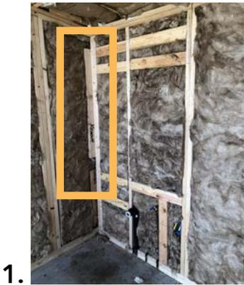
For Operable / Awning windows, drywall should return back to the window frame with a corner bead at the edge. We provide enough 4" MDF trim to serve as floor base and door casing, not as a window casing. **PRIOR EXPERIENCE IS RECOMMENDED.**
