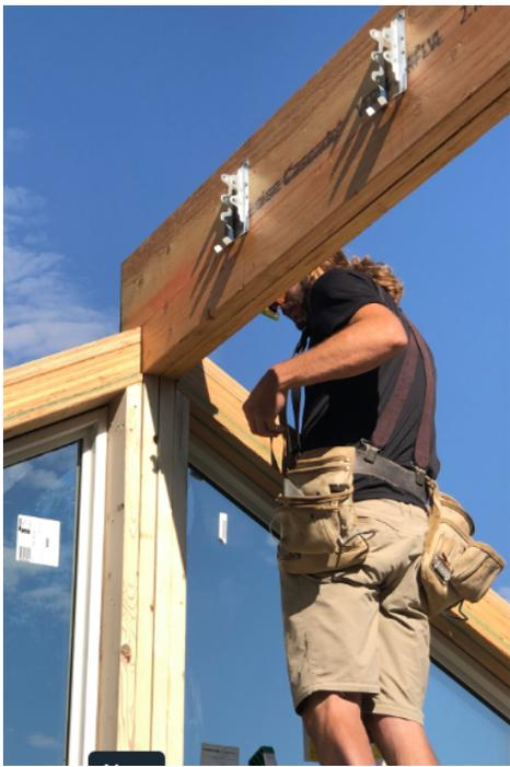
Once both ridge beam sections are in place, be sure to secure them together with construction screws. Typical pattern is three (3) screws at the mid-point between each rafter.
