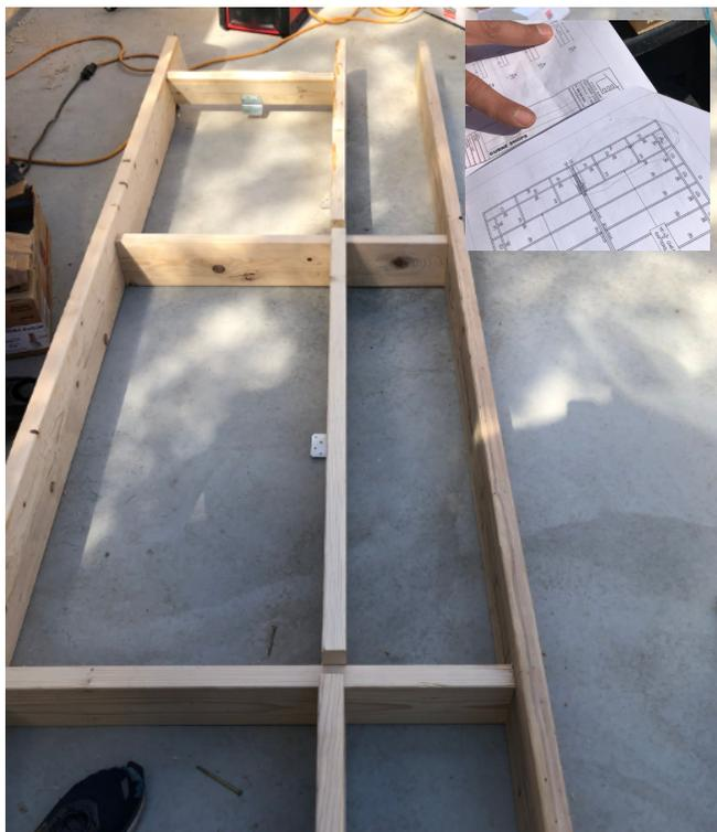
It is recommended to build the soffit overhang sections on the ground. Pre-install the A23 clips, and use a square tool to align the angled blocking with the pre-cut notches.
