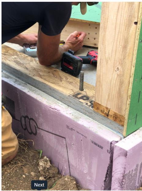
In some cases, hold-down embeds are called out. If this is the case, you will need to drill holes in the sill plate as well as in the bottom wall plate when you're standing wall panels. Carefully measure the center line of the embed, then use a 1" paddle bit to drill a hole for the embed to pass through.
