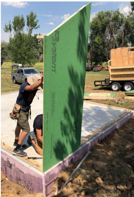
Note: Verify slab FF/FL prior to installing wall panels. You may need to shim wall panels (between sill plate and wall bottom plate) to maintain level walls. If this is the case, begin at the high point of slab.
