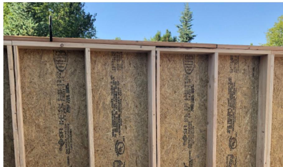
Install top plate on all four elevations. Top plate should be flush with top of wall panel.
