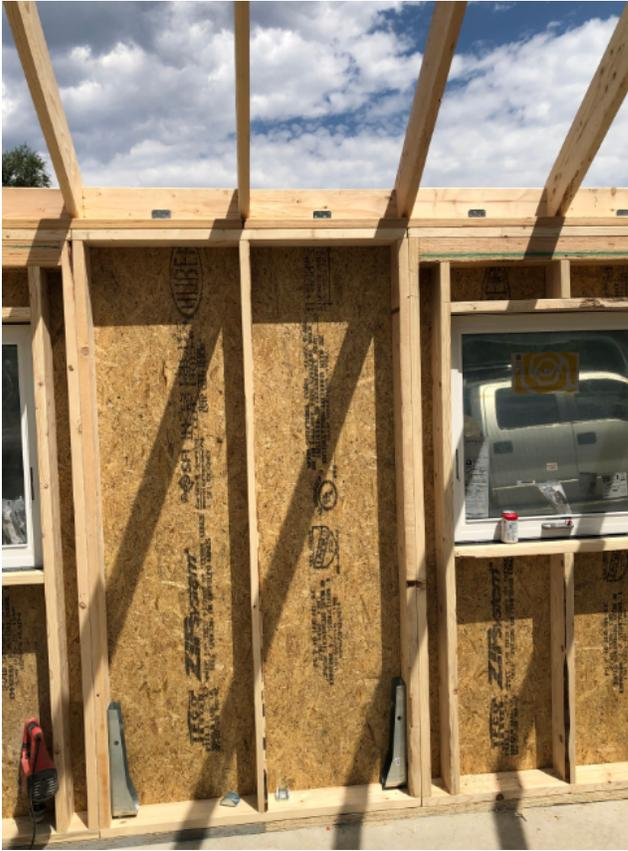
Rafters should align with wall studs. Timberlok screws are intended to replace hurricane clips, and are installed through the wall top plate into each rafter.
