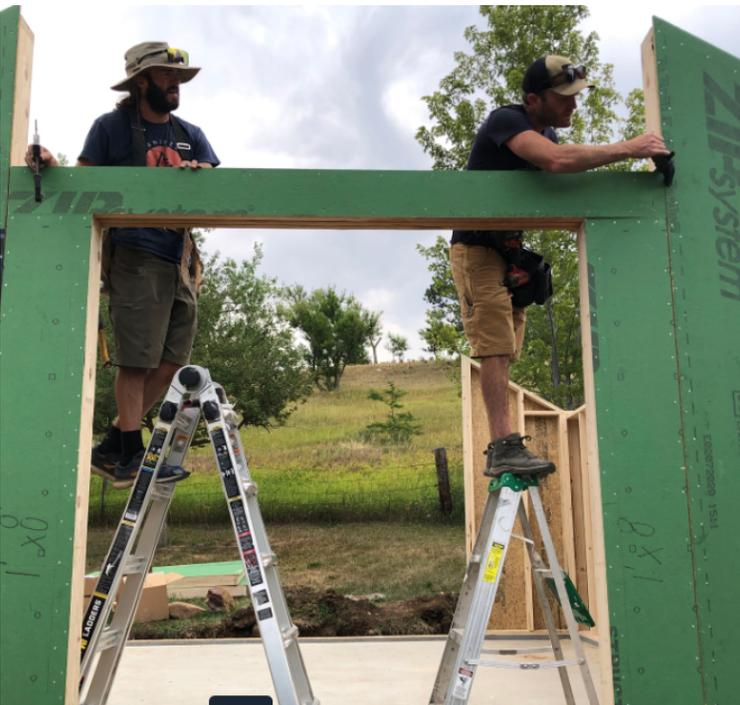
Use clamps if necessary, and verify the sheathing is flush between wall panels
