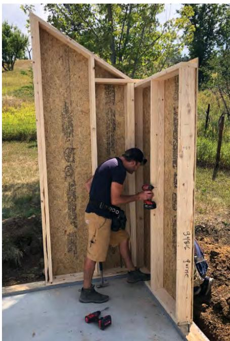
Continue standing side wall panels, ensuring the inside of overhang sheathing is tight to the sill plate.
