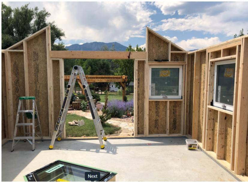
Interior view of installed wall panels and door header. It is important to make sure all wall panels are flush and plumb.
