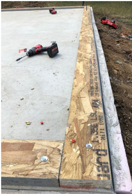
Pin sill plate to slab. Ideally, the sill plate is inset from edge of slab by 1/2" to allow wall sheathing to be flush with edge of slab.
