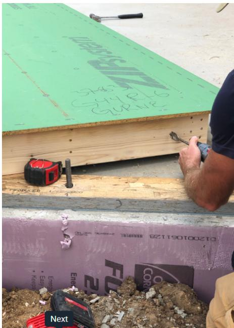
In some cases, hold-down embeds are called out. If this is the case, you will need to drill holes in the sill plate as well as in the bottom wall plate when you're standing wall panels. Carefully measure the center line of the embed, then use a 1" paddle bit to drill a hole for the embed to pass through.
