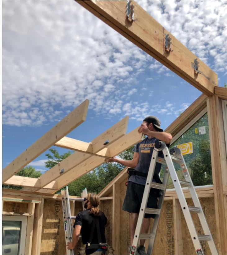
Guide each rafter section into place. You can run a screw through the top of rafter and into the ridge beam to secure it while working. Install rafter hanger nails in pre-drilled holes to permanently secure the rafters to the ridge beam and walls.
