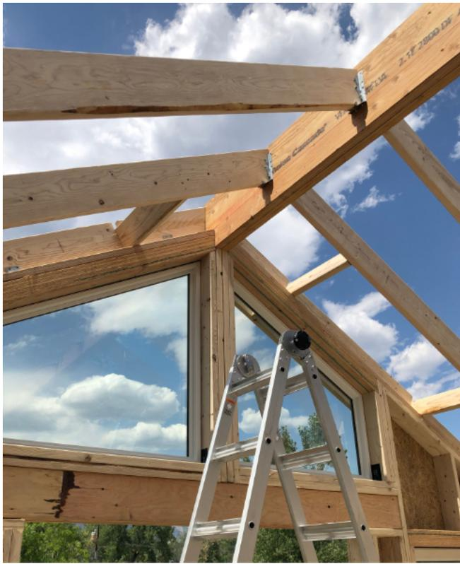
Final ridge beam and rafter assembly prior to installing roof sheathing.
