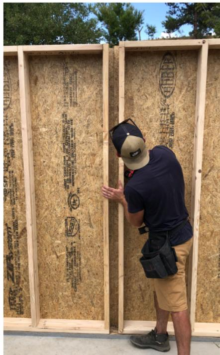
For panels with no windows or doors, the king stud gap will extend to the sill plate.
