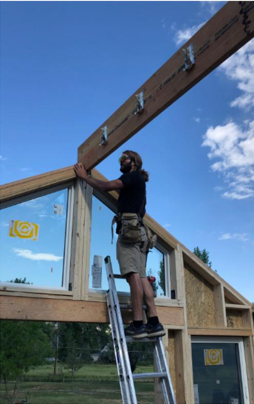
Once ridge beam is near the top of wall, rotate the beam and guide it into the pocket directly on top of the king stud.
