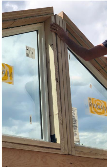
Install the partial-height king stud between window panels. This king stud will support the ridge beam.
