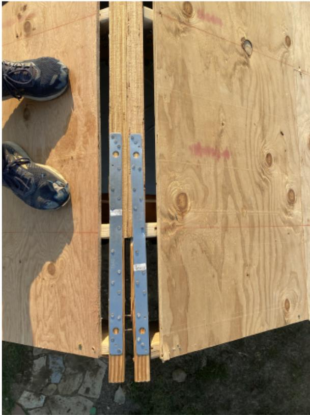
In some cases, straps will be used to secure the false ridge beam tails
