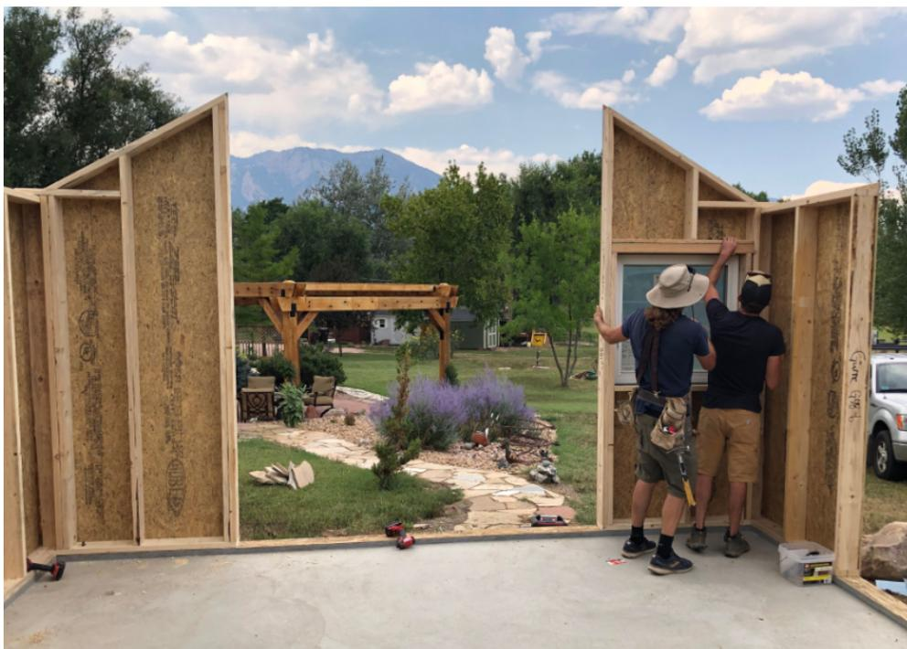
Continue standing wall panels. Install the front and back panels last.
