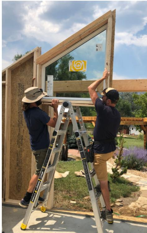
Carefully place trapezoid window panels on top of header. The top plate of the adjacent wall panel should be flush with the top of window header.
