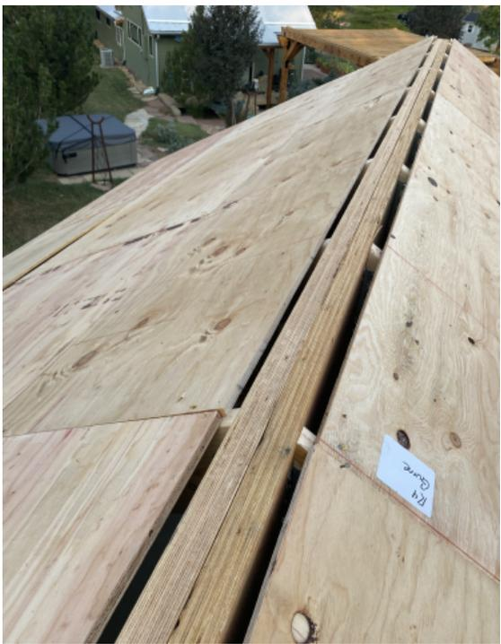
Sheathing should terminate below the ridge beam to allow for ventilation.
