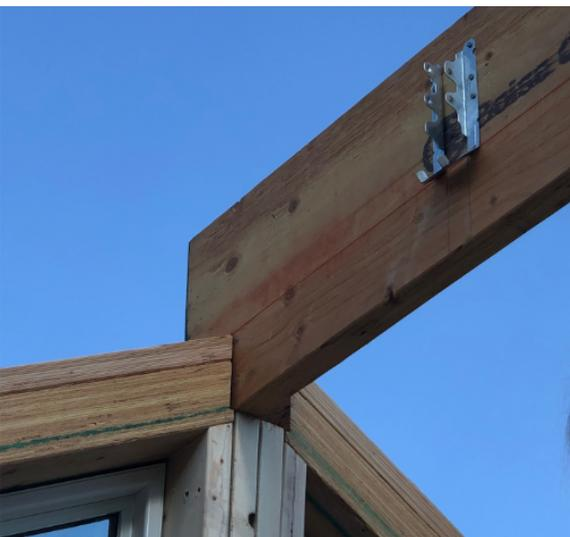
Whether the rafter hangers are pre-installed, or you install them in the field, ensure the bottom of rafter will be at the same elevation as the top of top plate on the wall.
