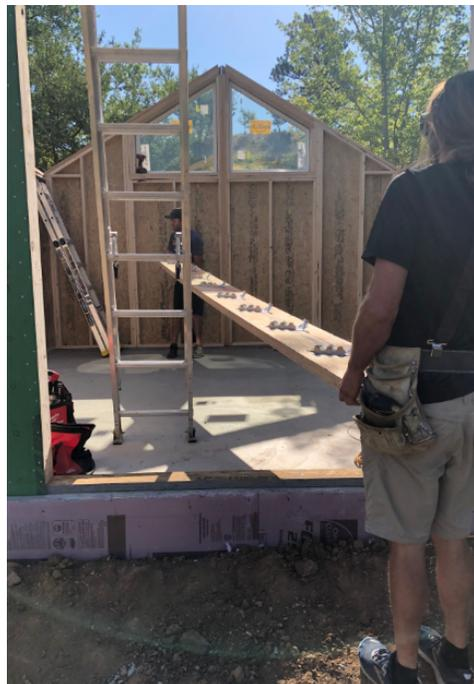
Carry ridge beam sections into structure, then lift into place. It can help to guide the beam along the top of gable wall panels instead of trying to lift it into place.
