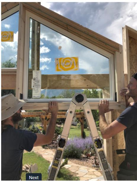
Carefully install remaining window panels. If necessary, temporarily screw the panel into adjacent studs to secure the window panel.
