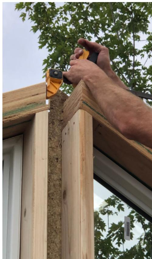
If necessary, use a reverse clamp to spread the opening apart to receive the king stud.
